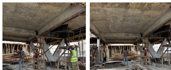
EICL Crescent today: first-floor slab complete, with the signature V-columns and structural frame in place.
